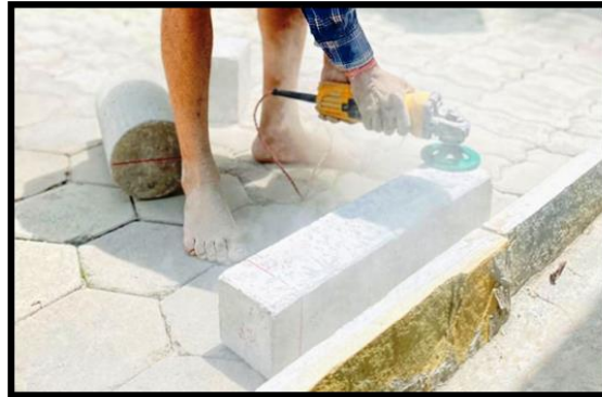
Figure 3: Surface Perparation of Beam Specimen
