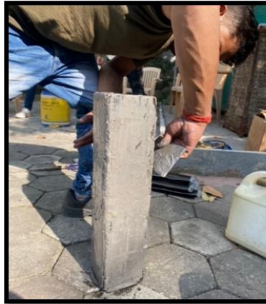
Figure 5: Application of Sealant
