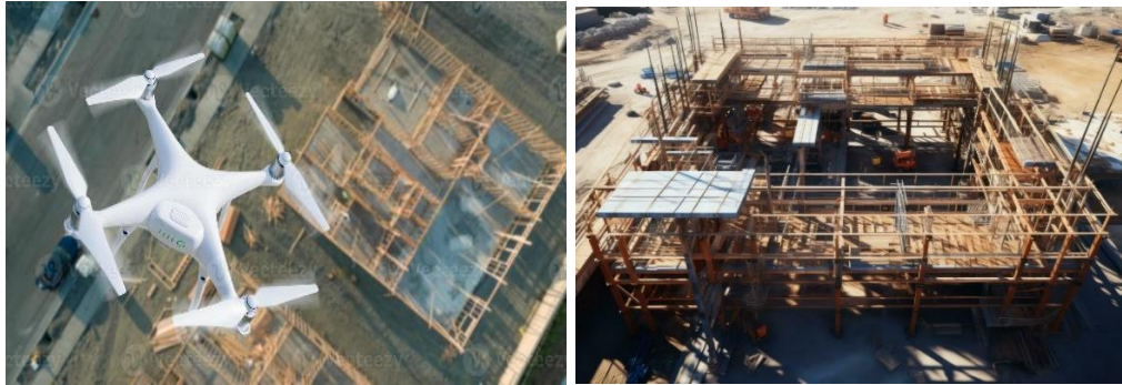
Figure 5: Drone construction Progress Monitoring
